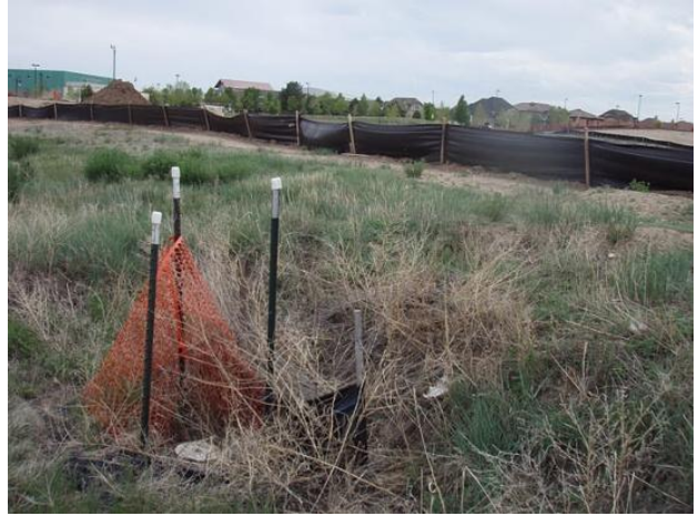
Photo 2: Snake habitat at the Lowry Wetlands site, currently under construction. The snake was found for several weeks living under the black plastic construction fence in the foreground.
